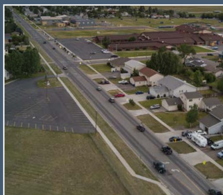
Urban roadways, like Jackrabbit Lane within the Belgrade Urban Area, typically include curb and gutter, bike lanes or bike boulevards, and sidewalks often separated by grassy boulevards.
