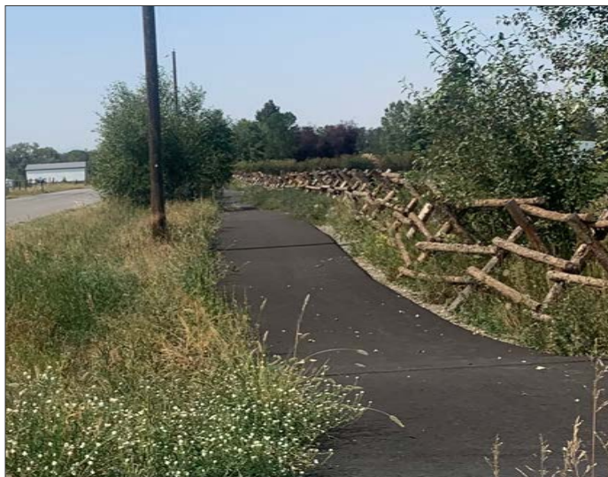
Good initial planning, proper design, and regular maintenance can help extend the life of shared use paths.
